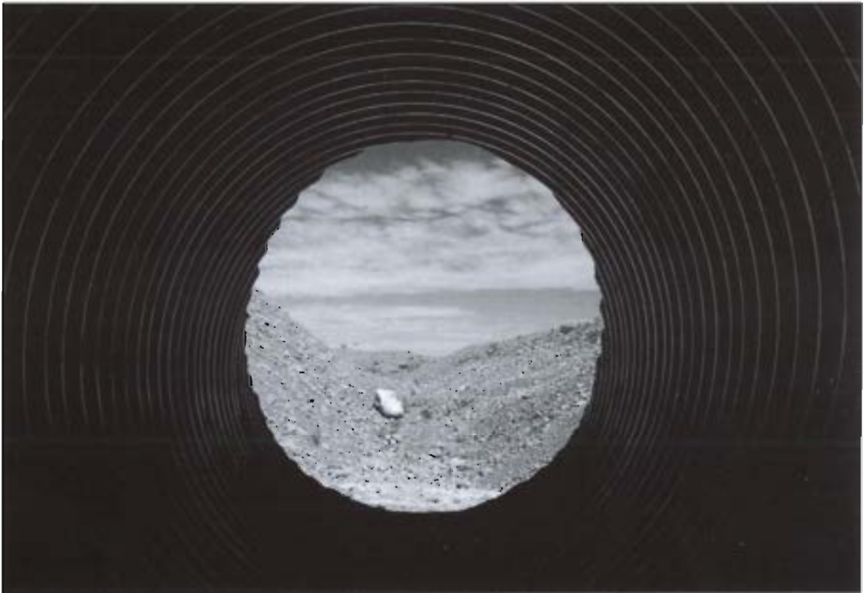
Through the culvert.
