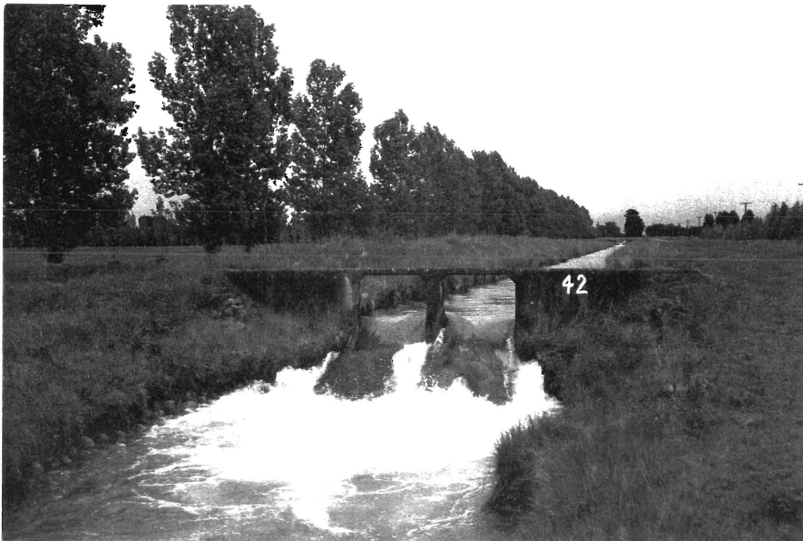
One of the many supply races which take water from the RDR to the farmers property
