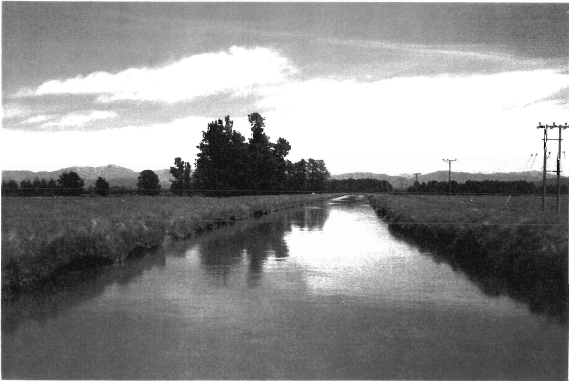
RDR supplying Irrigation water to 69,000 ha within Mid Canterbury
