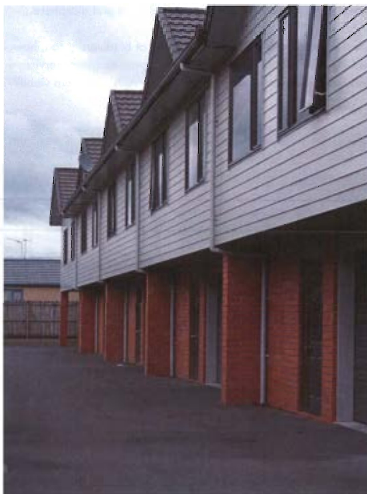
In-fill, high density housing replaces traditional homes with large gardens (Hamilton – Frankton).
