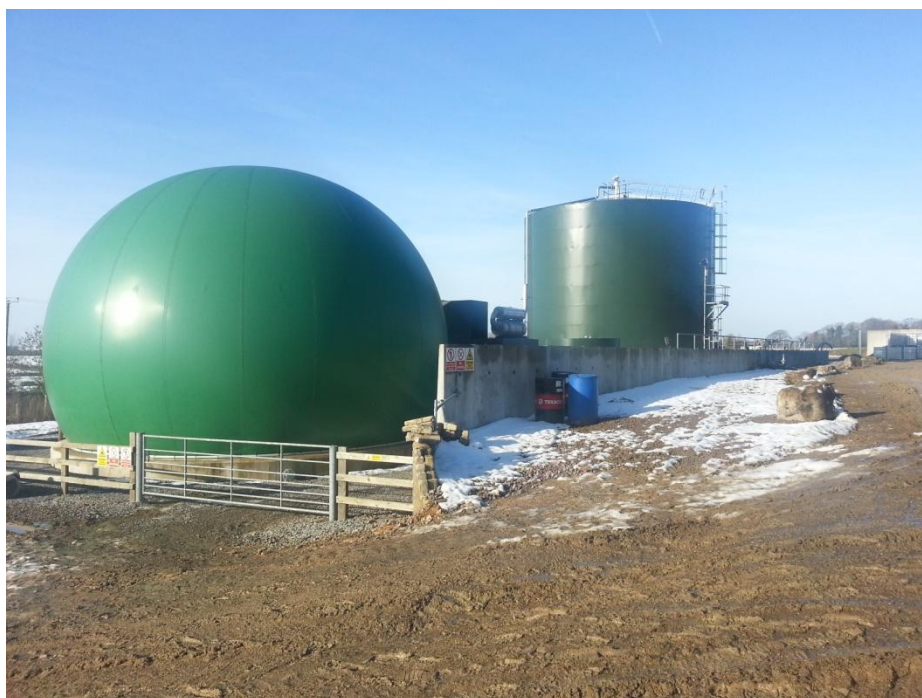
Figure 14: Kemble Farms Anaerobic digestion tanks
