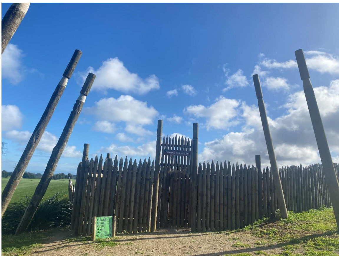
Figure 3: A traditional tuwhatawhata [palisaded] pā named Ōhaurai which has been constructed on a farm near Hāwera to protect a propagation house (Rongo-marae-roa) and a smaller shade house (Tane Mahuta).
